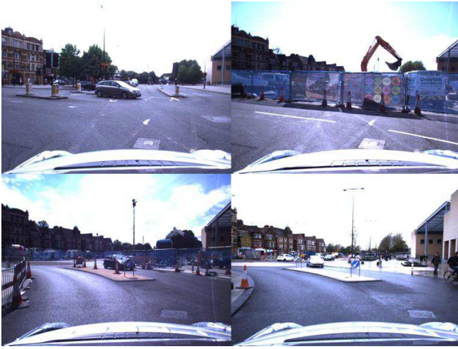
Fig. 7. Structural change in the environment over time. The original intersection (top left) was redeveloped over a period of months, resulting in redirection of traffic during construction (top right, bottom left). The final intersection (bottom right) has a completely different road layout, replacing traffic lights with a roundabout.
