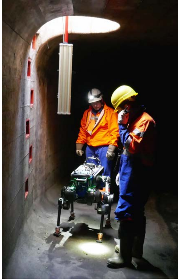
(a) ANYmal setup in the sewer
